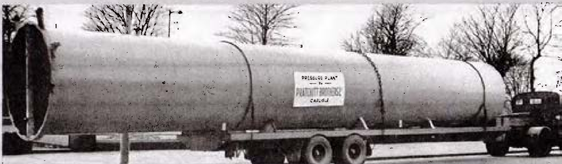
▼ Pressure Impregnating Cylinder 7' 6" dia. x 53' long en route to site
